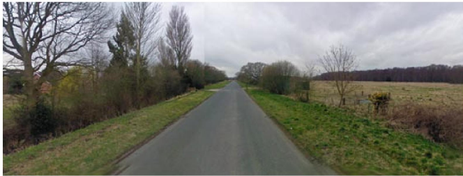
View 3. View looking east along York Lane
